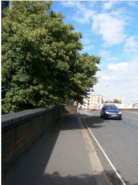
Photo 2.7: Looking north along Central Bridge
