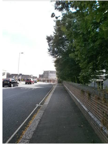
Photo 2.8: Looking south along Central Bridge
